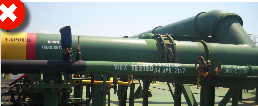
The medium used for the test should be also stenciled
