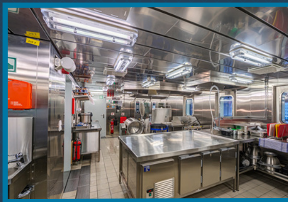
'Galley Preparation for P.S.C. inspection'
